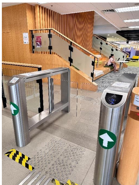
Access gate at G/F
