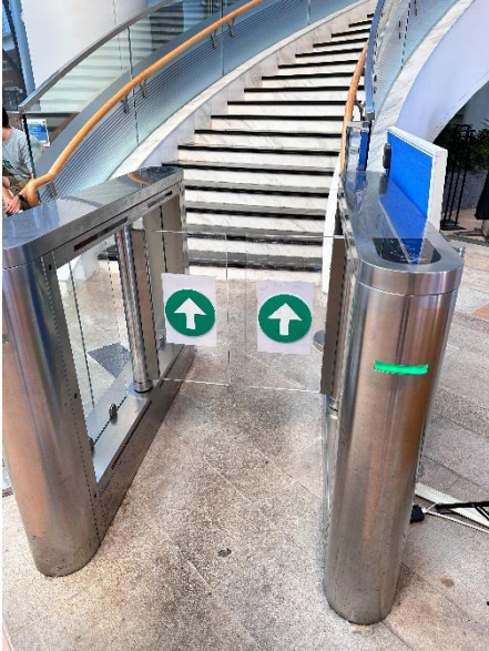
Access gate at G/F
